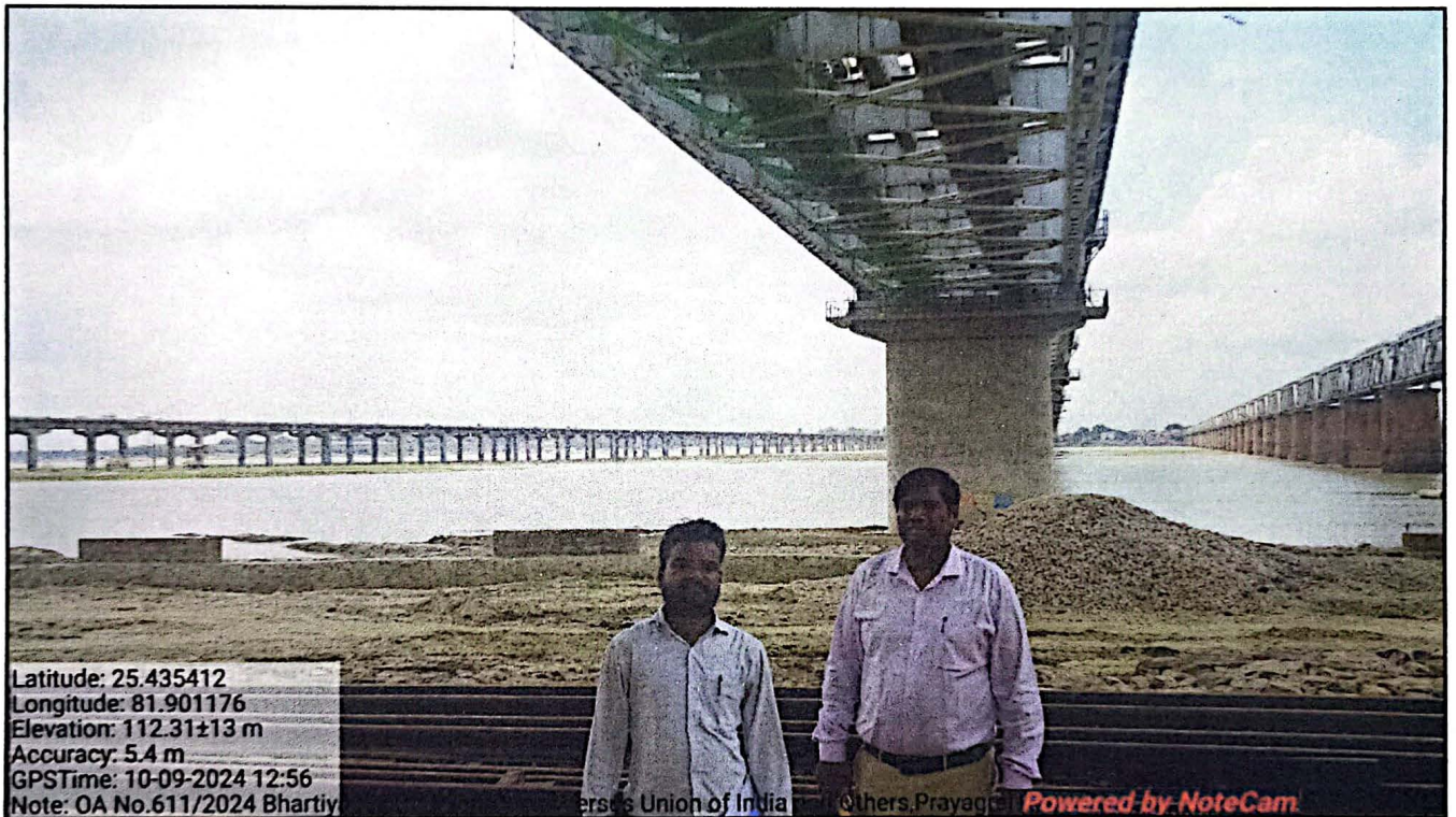
Photographs showing newly constructed Rail bridge over River Ganga near pier no. 01 towards Jhunsi, Prayagraj on dt. 10.09.2024.
